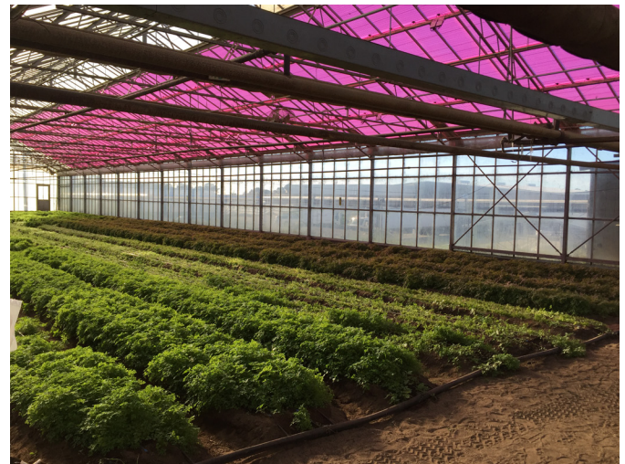
Figure 4. Solar greenhouses in Canada fitted with Soliculture's WSPVs, technology developed by UCSC. Source: Soliculture
