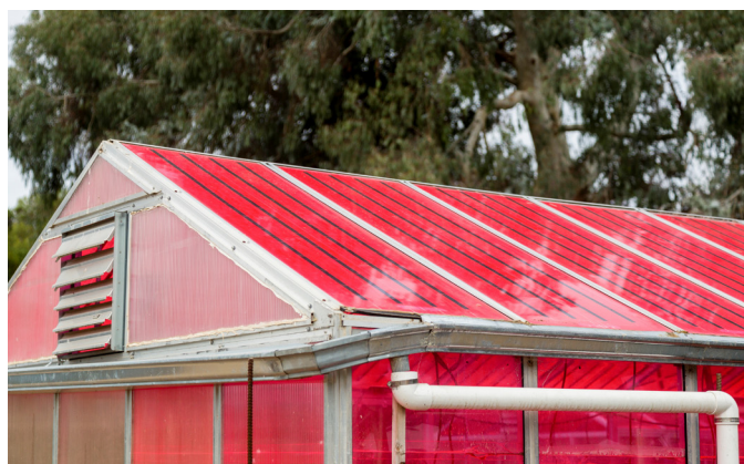
Figure 3. UCSC's pilot solar greenhouse with WSPVs. Source: Nick Gonzalez, UCSC
